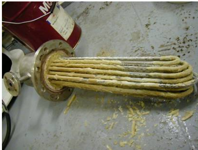
Heat exchanger aboard the Norsky, 12 February 2006
